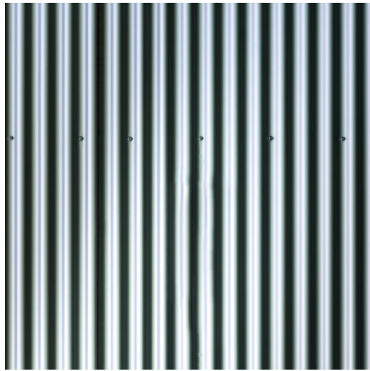
Al01 Selected galvanised corrugated steel cladding. To exterior facade.
